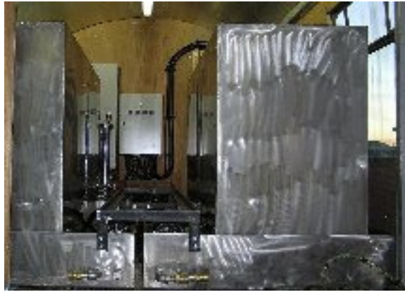
Picture 1.3. Herbicide storage tanks.
